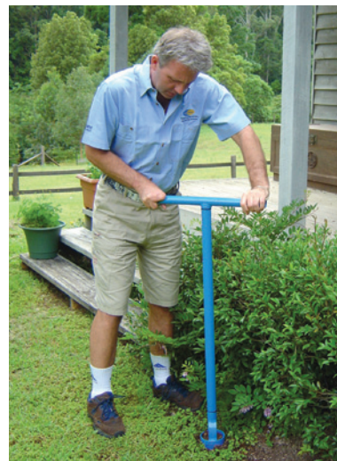
Using auger to place Exterra Station.
